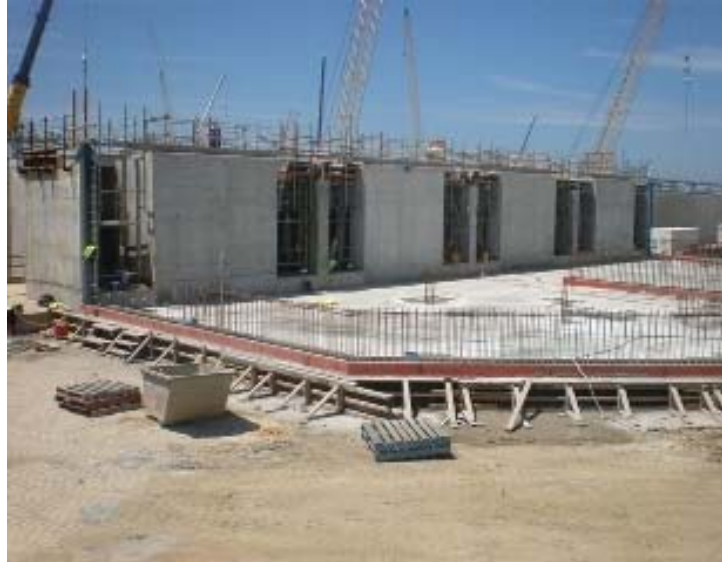
Ausform's concrete water retaining structures
