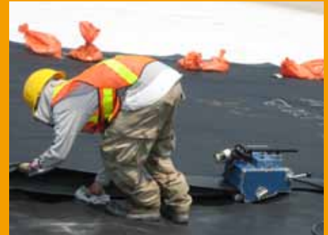
Installing HDPE lining
