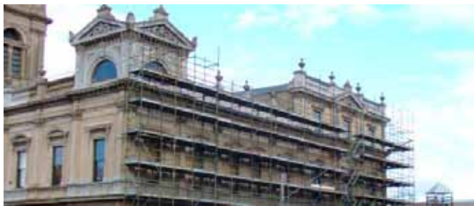
Nicholson Construction renovation works on the Ballarat Town Hall
